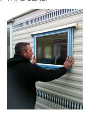
ONCE THE WINDOW IS FULLY IN, THE PERSON ON THE INSIDE SHOULD FIT THE INTERNAL TRIM TO THE SEARRTED PART OF THE PROFILE, USING THE NYLON FACED HAMMER THE PERSON SHOULD THEN HAMMER IN THE TRIM, THUS PULLING THE WINDOW IN TIGHT, REPEAT THIS FOR ALL 4 SIDES, ONCE IN IF THE WINDOW OPENS, OPEN THE SASH AND SCREW 2 FIXING SCREWS, 1 PER SIDE THROUGH THE FRICTION STAY (HINGE) WERE A SCREW HOLE IS SHOWING. TAP ON THE 4 MOULDED CORNERS TO LEAVE AN INTERNAL DECORATIVE FINISH.
